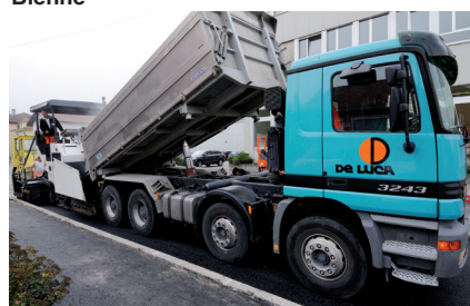
Route cantonale, Bévillard
